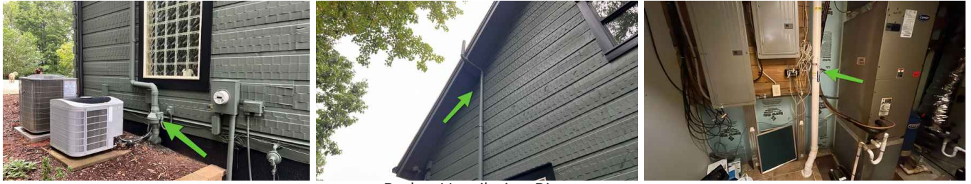
Radon Ventilation Pipe
