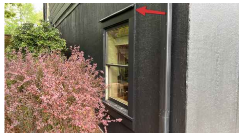
No flashing with wood rot at window
